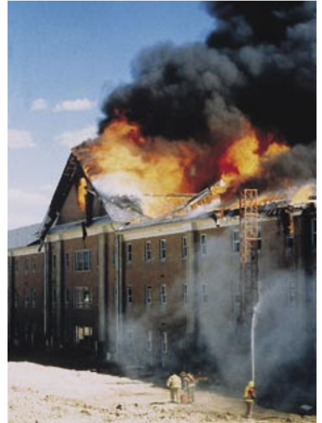
Fanned by high winds, a fire raged in the wood roof framing of this mostly precast concrete structure of the Oaks at Medina continuing-care facility in Medina, Ohio. The fire burned for four hours, leaving some concerned about how extensively the building was damaged and how long it would be before the building could be repaired.
